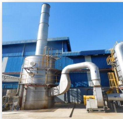
YMI Blower and Wet Scrubber for gas Neutralization
