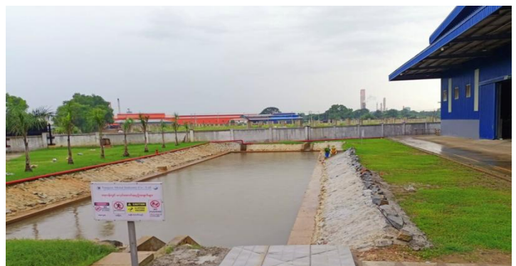
Receiving/ Storage tank for waste water collection at YMI
