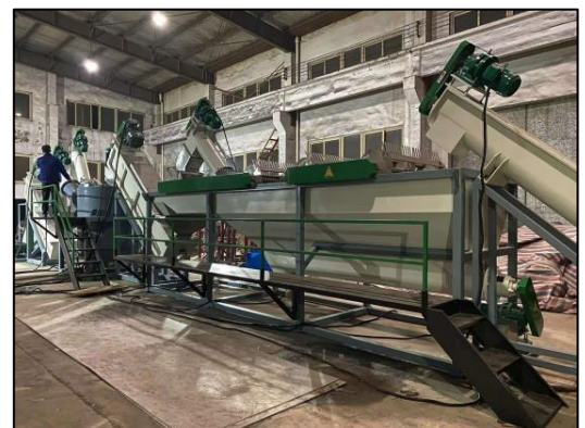
Plastic Recycling Plant at YMI
