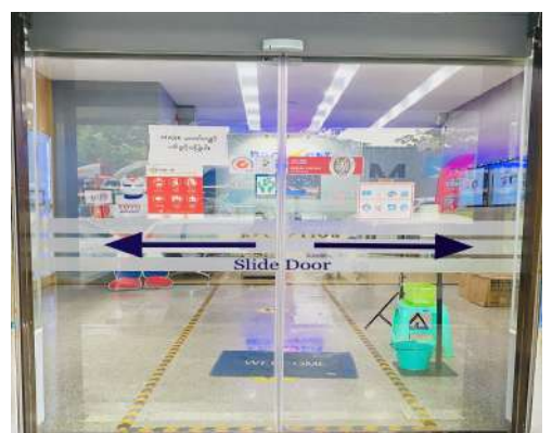
Installation of auto slide door
